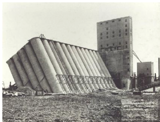
Transcona Grain Elevator, Canada (Oct. 18, 1913) - Typical Example of
